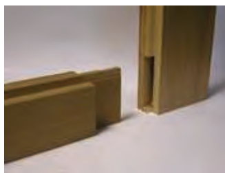
Mortice and tenon joint
